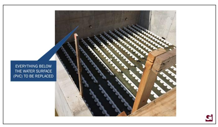
Construction of an Above-Grade Aeration Piping System Replacement of the Existing Ceramic Diffusers with EPDM Diffusers
