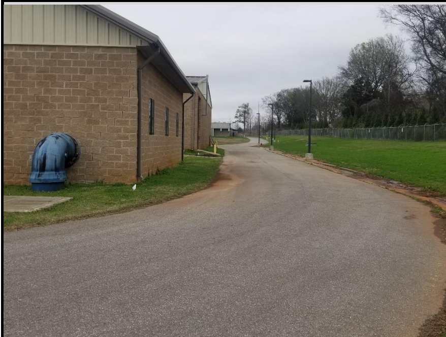
Description: Viewing north of service road along east side of the Filter Building
